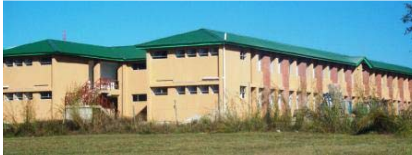
Fig. 1 – Almost completed Student Hostels
